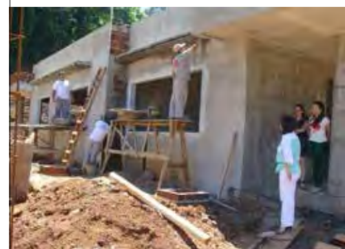
Social Assistance Reference Center under construction in Seara
